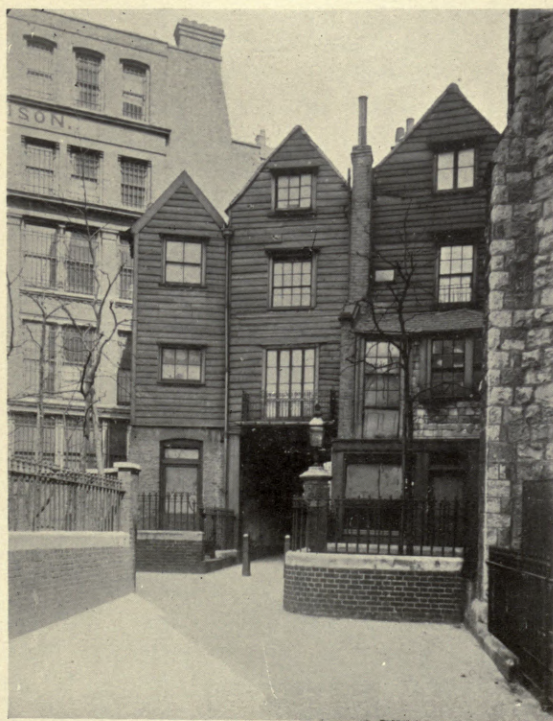
OLD WOODEN HOUSES AT CRIPPLEGATE (RECENTLY DEMOLISHED).
